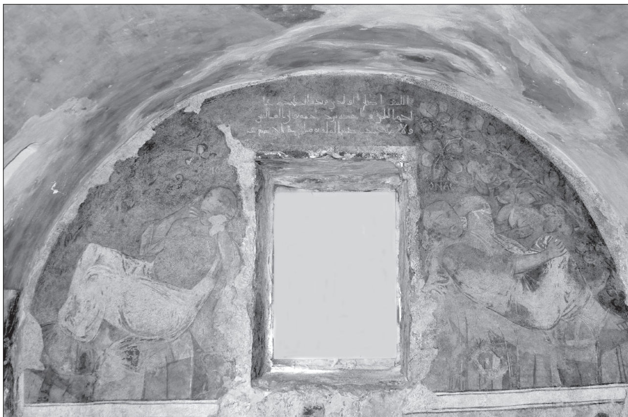
4. Representation of Jonah on the lunette of the south wall (main hall, west aisle).
